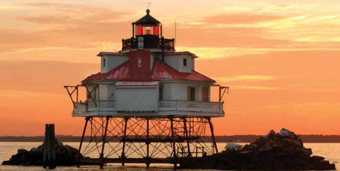
Thomas Point Lighthouse, in the Chesapeake Bay off Annapolis, Maryland.
